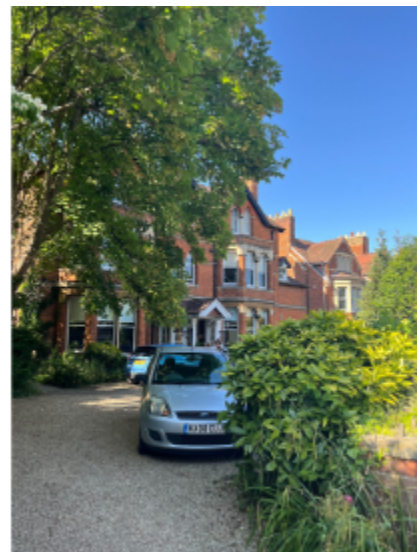
3 Bardwell Rd. This is St. Clares' academic building.
